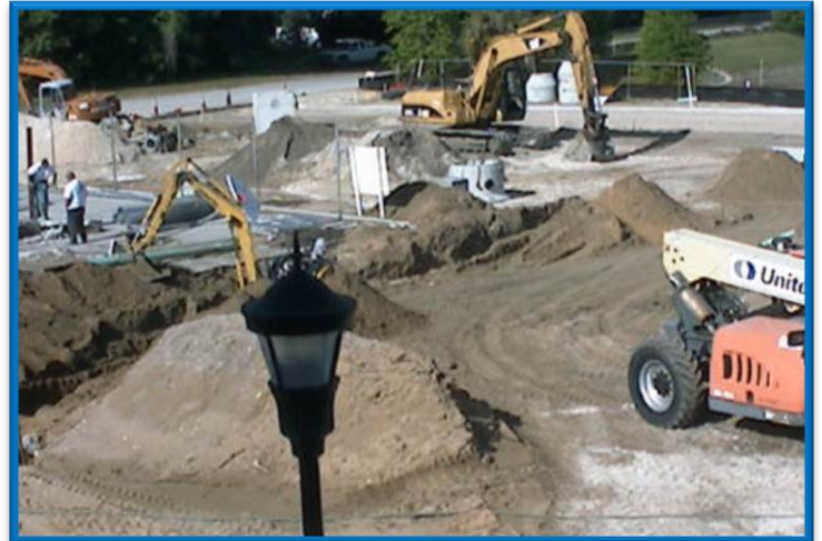
Construction in process
